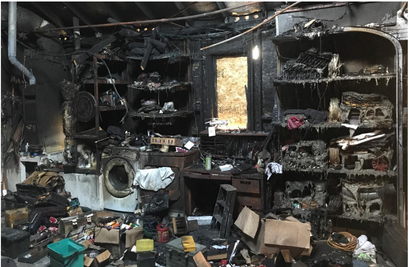
Residential garage fires typically consume large quantities of plastics, PVC, and synthetic materials.
