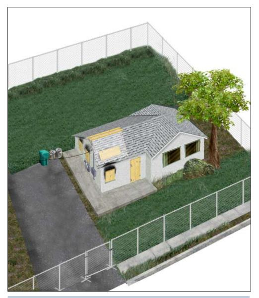
Board-Up of Windows, Doors and Roof Hole. Lot secured with Perimeter Fencing.
